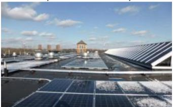
CDM Smith designed a photovoltaic (PV) system at the Water J Sullivan Water Purification Facility, which will supply power on-site for water treatment operations. Photo courtesy of CDM Smith.
